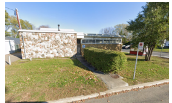
Location of 3rd work: REIP pumping station (intersection of Shamrock and Northcote streets).
